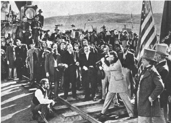
UNION PACIFIC To shoot this drama of the growth of American transportation, De Mille bought or rented enough equipment to start a short railroad line. Painstaking historical research went into this 1938 production
